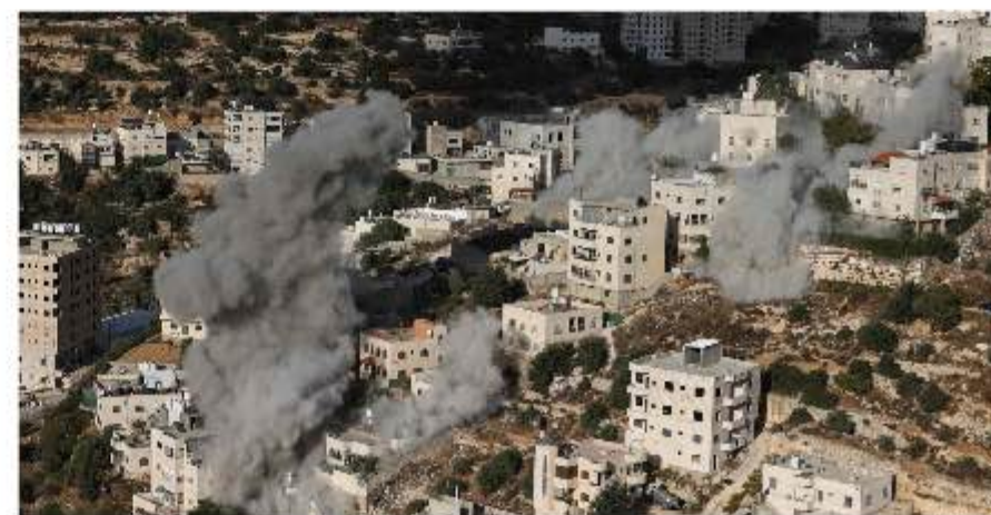
Smoke rises as the Israeli military demolishes the homes of the two Palestinian gunmen who killed two Israeli soldiers at a West Bank checkpoint the previous week, in the Israeli-occupied West Bank city of Hebron, on Friday
