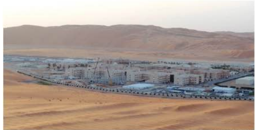
Photo by Arab News Saudi Aramco's Shaybah oil field in the Eastern Province
