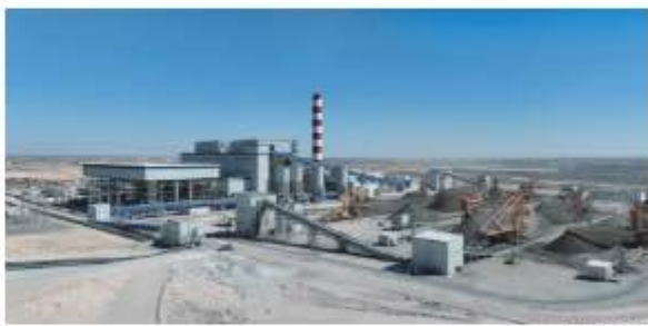
Attarat Power Company has won two awards at the 2026 Asian Power Awards in recognition of its pioneering oil shale-fired power generation project
