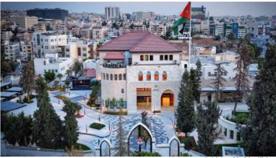
Aerial view of the Prime Ministry
