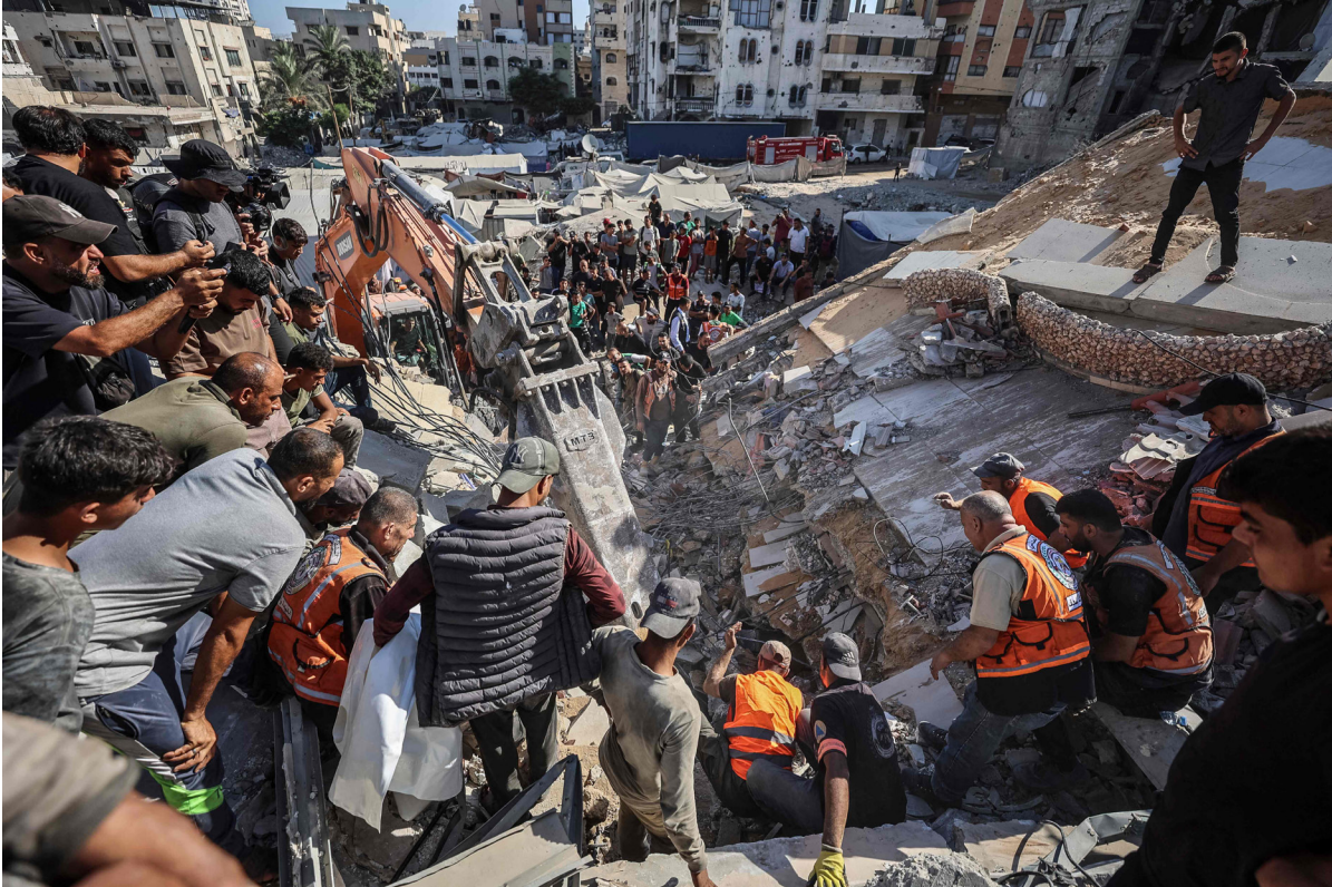
AFP photo Rescuers excavate rubble to retrieve bodies from a collapsed building in the Tal Al Hawa area of Gaza City on Wednesday
