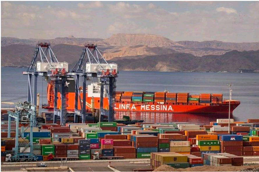
Aqaba Container Terminal
