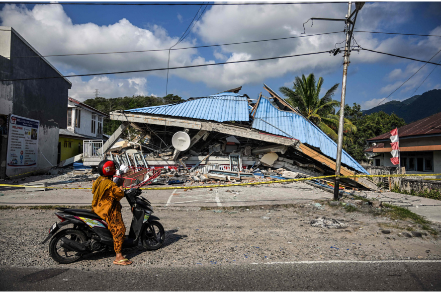
A motorbike stops next to a collapsed building following a 7.7-magnitude earthquake in Borong, East Manggarai, East Nusa Tenggara on Sunday
