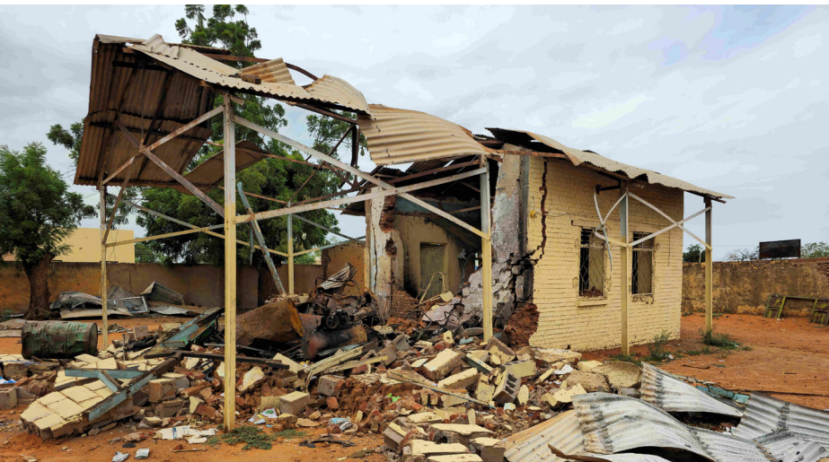
This photo shows a general view of a destroyed building after the Rapid Support Forces targeted several civilian facilities in Al Rahad Abu Dakna located on the national highway linking Kosti and El Obeid, on Saturday
