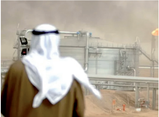
An employee of the Kuwait Oil Company looks at 25 January 2005 the Gathering Centre No.15 of Al Rawdain field, 100 kms north of Kuwait City
