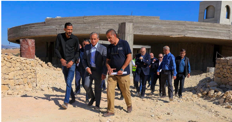
Photo courtesy of Prime Ministry
