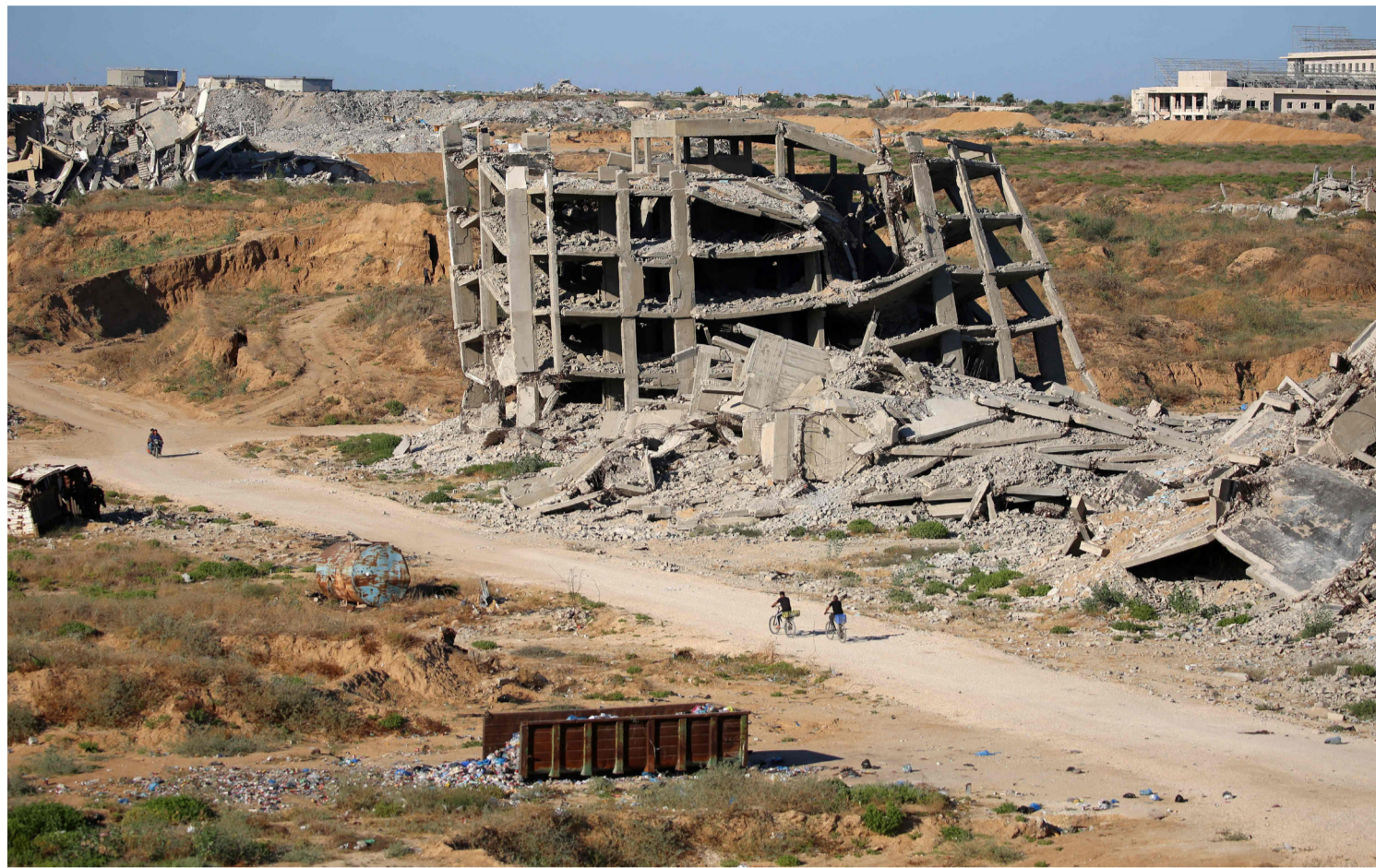
Men ride bicycles past a heavily-damaged building at the Nuseirat camp for Palestinian refugees in the central Gaza Strip on Friday
