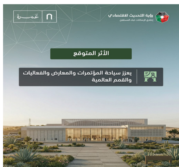
The Amra International Convention and Exhibition Centre would serve as a major venue for exhibitions and large-scale events in the Kingdom and forms part of the first phase of the Amra City development
