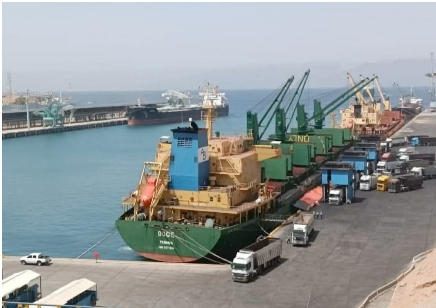
The Aqaba Development Corporation (ADC) says on Monday that it had commenced detailed studies and designs for a new JD45 million oil derivatives pier
