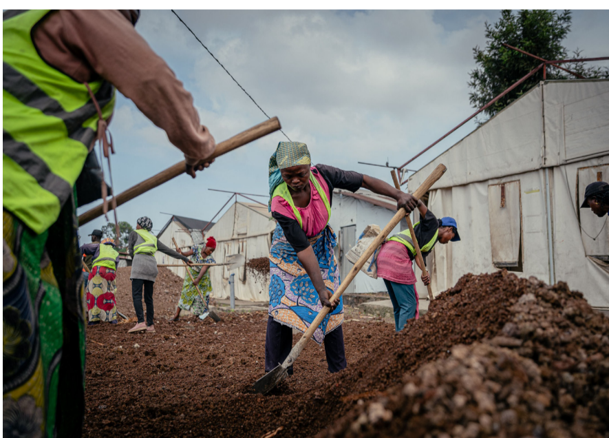
Workers from Kanyaruchinya, in Nyiragongo territory, take part in sanitation, renovation, and levelling work at the former Ebola treatment centre, in Goma on Tuesday
