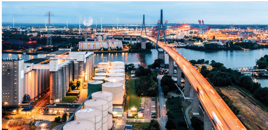
An illuminated power station, flyover and Hamburg docks
