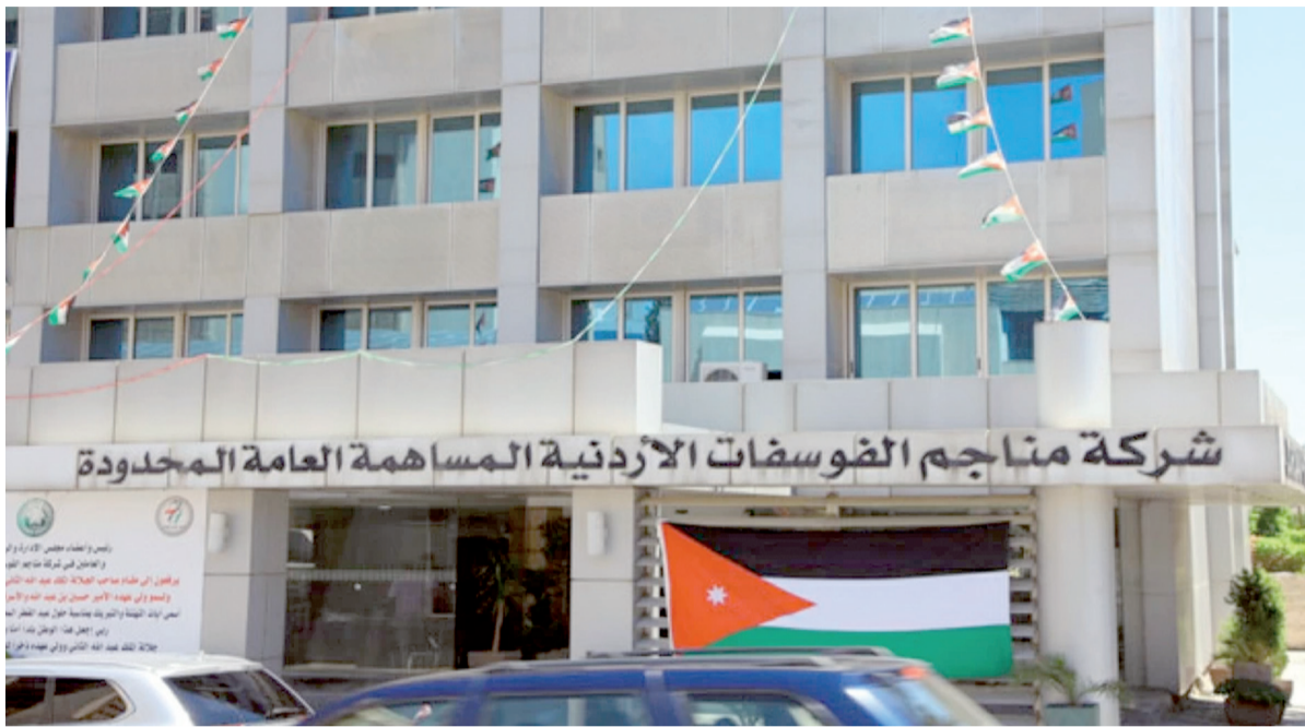
The General Assembly of the Jordan Phosphate Mines Company has approved the board of directors' report on the company's 2025 operations and its future action plan during its 72nd ordinary meeting
