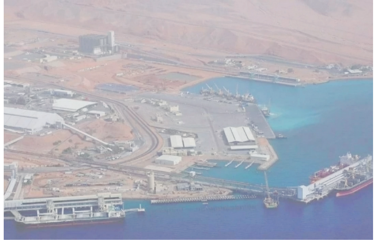
Aqaba Ports Company announces on Saturday the completion of a project to upgrade two mobile cranes, with the German manufacturer Konecranes Retrofit, at a cost of JD600,000
