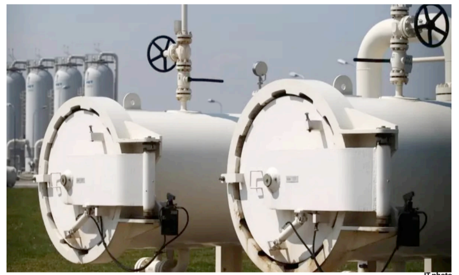
The gas compression plant (Jordan chlorine) that is currently under construction in the Risha region
