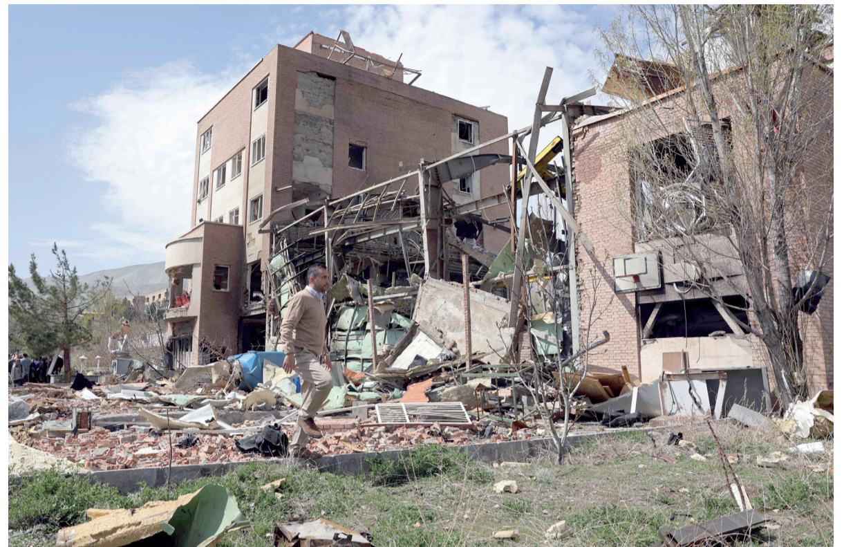
A man walks past the damaged building of the Shahid Beheshti University following a strike, in Tehran on Saturday
