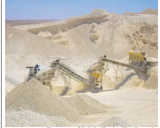
Al Wadi Al Abyad phosphate mine in the Karak Governorate, located some 115 kilometres southeast of Amman
